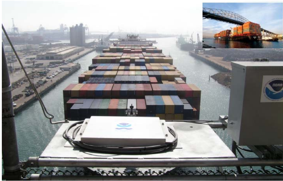
NOAA's air gap sensors allow large ships to pass safely under bridges
