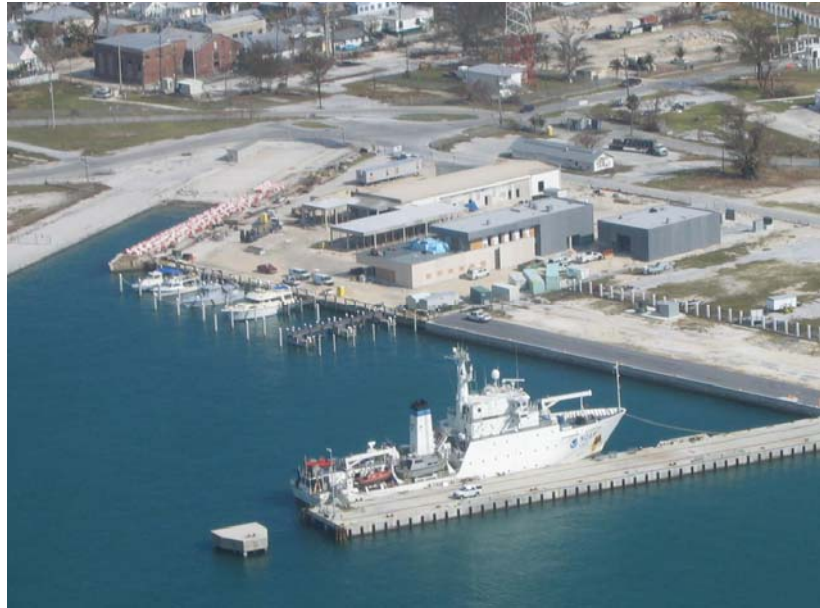
The Dr. Nancy Foster Florida Keys Environmental Complex, currently under construction, will feature 6,000 square feet of interactive exhibits on the Florida Keys.
