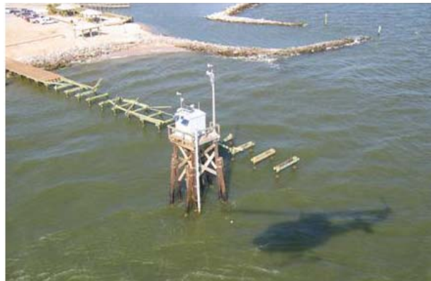
NOAA's "hardened" NWLON station in Dauphin Island, AL withstood the forces of hurricane Katrina, while the pier it was attached to was destroyed
