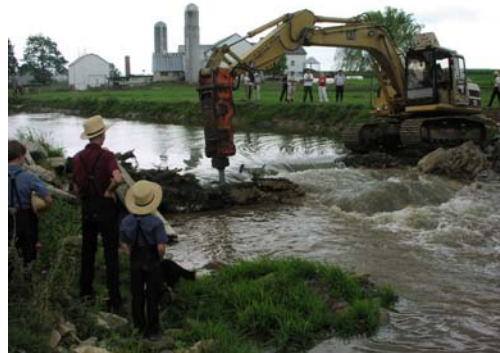
Mill Creek dam removal
