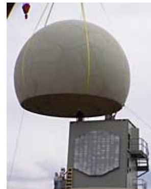
Installation of the SPY-1A antenna and radome on the NWRT
