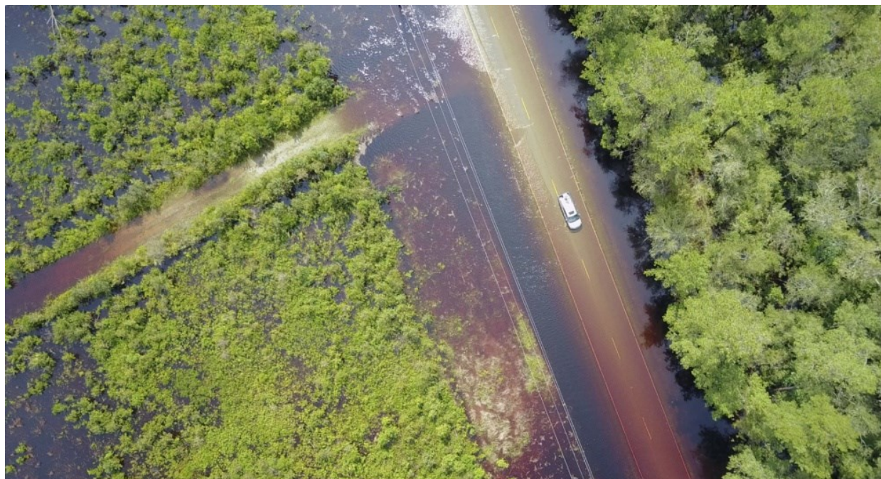
Flooding after a hurricane can sometimes be the most damaging part of the event. Roads can be cut off by flooding, as in this photo of flooding caused by Hurricane Florence in Ringlewood, North Carolina. The Southeast and Caribbean region has been working to increase awareness of roles and responsibilities for NOAA staff during an event—making everyone safer. (Photo Credit: Air National Guard)
